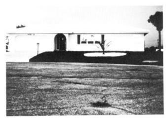
Figure 4.1. Elevation by Earth Fill
