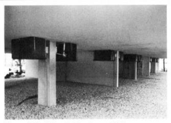
Figure 4.49. Elevated Condenser Units
