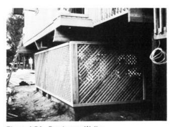
Figure 4.54. Breakaway Walls
