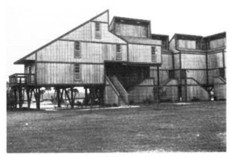
Figure 4.4. Elevation by Posts
