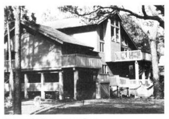
Figure 4.3. Elevation by Posts
