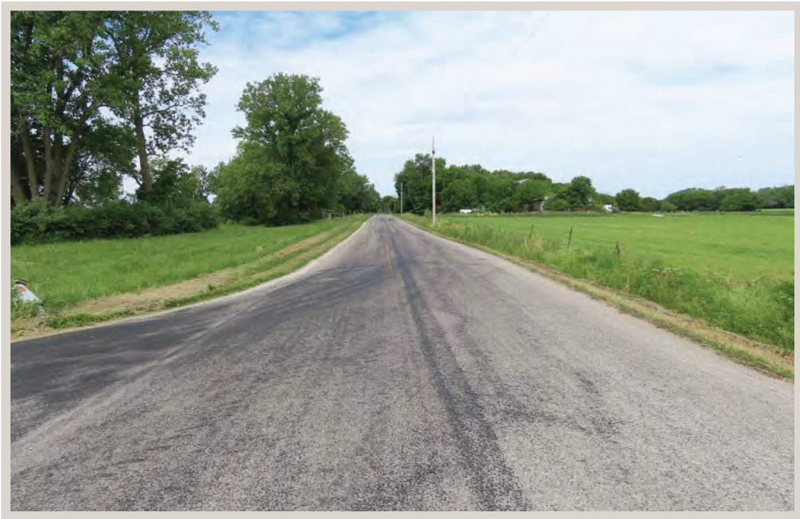
Photo 3: Looking west along E. County Road 200 South from County Home Road.
