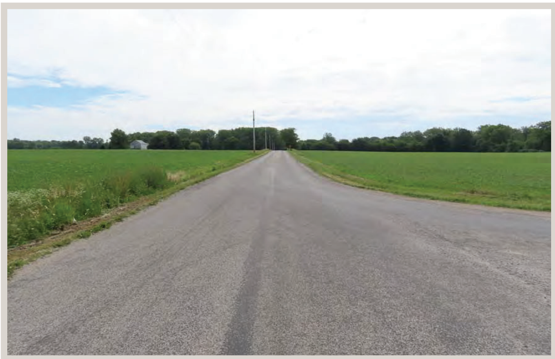
Photo 4: Looking east along E. County Road 200 South from County Home Road.
