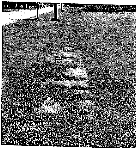
Grade D – Multiple Major Deficiencies: For instance, the sidewalks shown here are too narrow, they have joint displacements, rough/cracked surfaces (or stones), and gaps making it likely impassable by wheelchair, though a fit walker could still navigate them.
