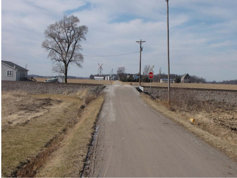
Photo 3: CR 250 South – Railroad Crossing Facing West
